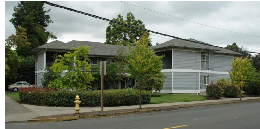
Mill Street Apartments (credit to St. Vincent de Paul and Apartments.com): 10 units of housing at 50% AMI; 5 lower units share a kitchen, and 5 upper units share a kitchen. Each unit has its own bathroom.
