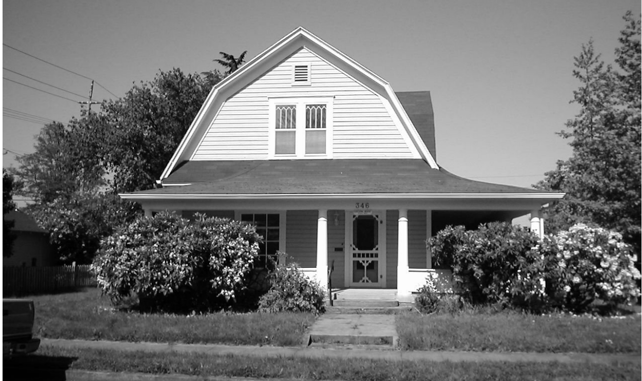
Figure 34. Dutch Colonial located at 346 7th Street. (Photo by D. McCormack, 2003)
