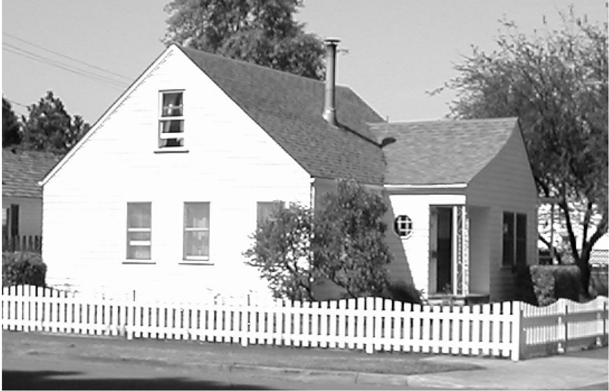
Figure 36. Minimal Traditional Style located at 757 'E' Street (Photo by D. McCormack, 2003)
