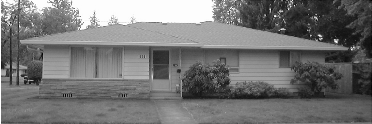
Figure 38. Ranch Style located at 757 'D' Street (Photo by D. McCormack, 2003)
